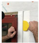
Adhere the tape from sill down and over the ThermalBuck and onto WRB.
