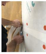
Press AND roll the tape to ensure a good air & water seal.
