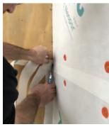
Roll the tape to ensure a good air & water seal.
